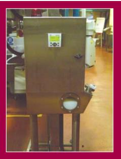
TO THE LEFT IS THE **DLAC DLU5000** CENTRAL CONTROL UNIT CONSTRUCTED IN STAINLESS STEEL WITH IP65 PROTECTION CLASSIFICATION. THE CENTRAL UNIT CONTAINS AN INTEGRAL 1 1 LITRE LUBRICANT STORAGE RESERVOIR POSITIONED BELOW.
